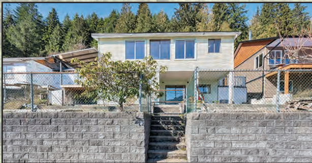
Oceanview Family Home: Attractive 2-story home with ocean and mountain views in Tahsis. 4 bedrooms, open concept living space, good storage. Two patios, large windows, wood features throughout. Shop with power and vehicle access. Terraced property, with firepit on the upper level. Lane and road access. Short walk from marina. West coast Vancouver Island. $289,900
