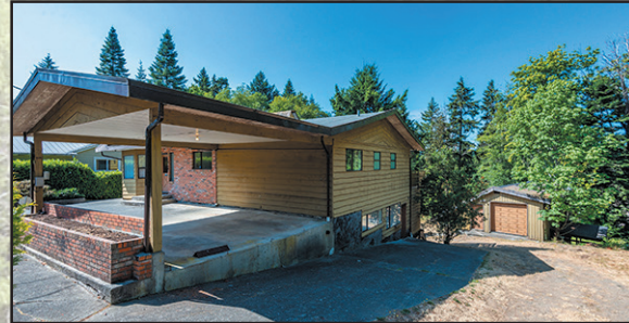
Rare Campbell River Property: Half acre in town, 4560sqft home on three levels and a large, two-story workshop/garage. Lower back yard with walkout access from the home, and undeveloped natural space behind. Built by a local developer in the 80s for his personal property, the home and shop are constructed to the highest standards of the time. $974,900
